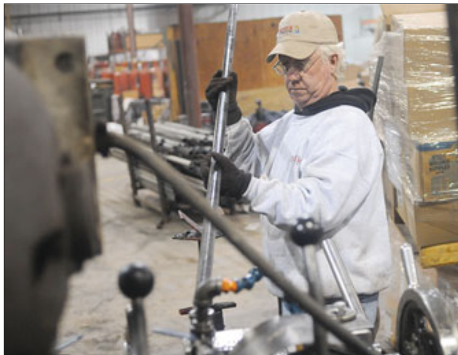
Richard McClain threads a one-inch pipe that is used for sprinkler systems at Premier Fire Protection Inc. in Paducah.
